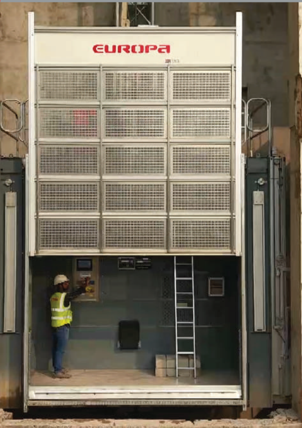
India's tallest 305-meter height installation of a 3-door (C-type) Customized Europa YHX Hoist as on December 2024
